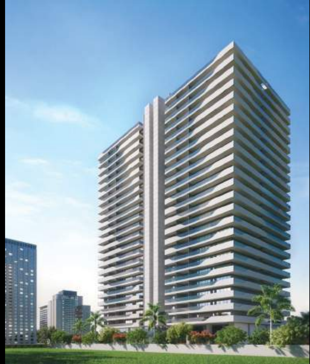
View from the north-east side
